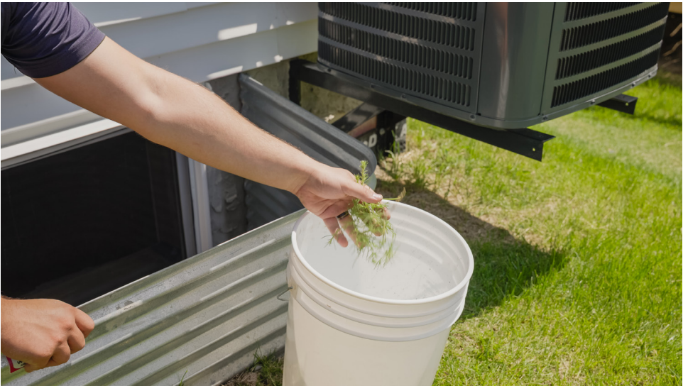
Image Description: Removing debris from window well.
