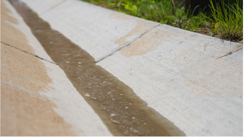
Image Description: Concrete swale along property line.
