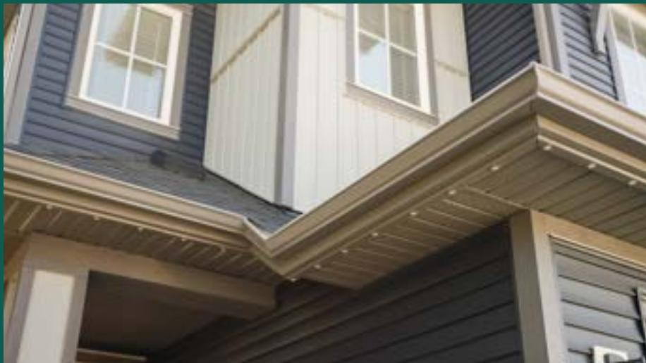
Efficient rooftop drainage will help you keep your basement dry. Eavestroughs move water to downspouts and away from your home or from your downspout to the drain, below ground. During heavy rainfall, this drainage system can move hundreds of gallons of water in a single day so it's important that eavestroughs are sloped towards the downspouts and are clear of debris. Surface particles from asphalt shingles are often washed away by rain and settle in the eavestroughs, reducing their efficiency.
